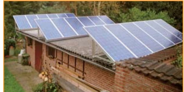
Flatroof-mounted System 3.0 kWp
