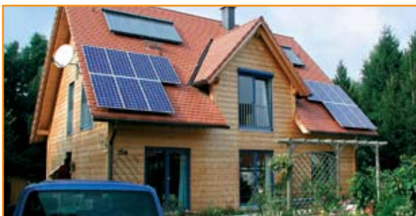
Roof-mounted System 2.1 kWp
