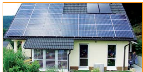
Roof-mounted System 8.0 kWp
