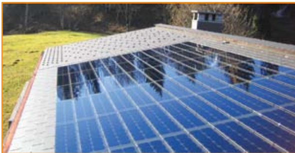
Roof-integrated System 5.6 kWp
