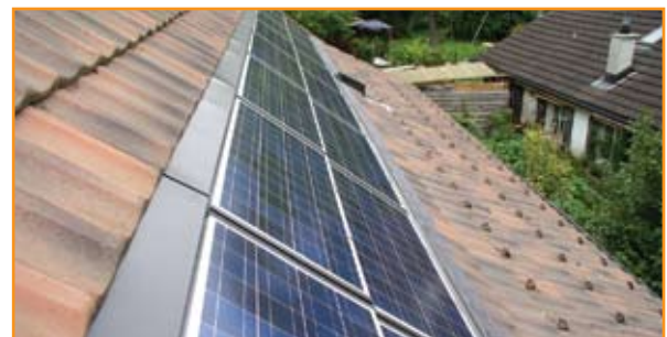
Roof-integrated System 3.2 kWp
