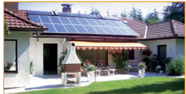
Roof-mounted System 3.0 kWp
